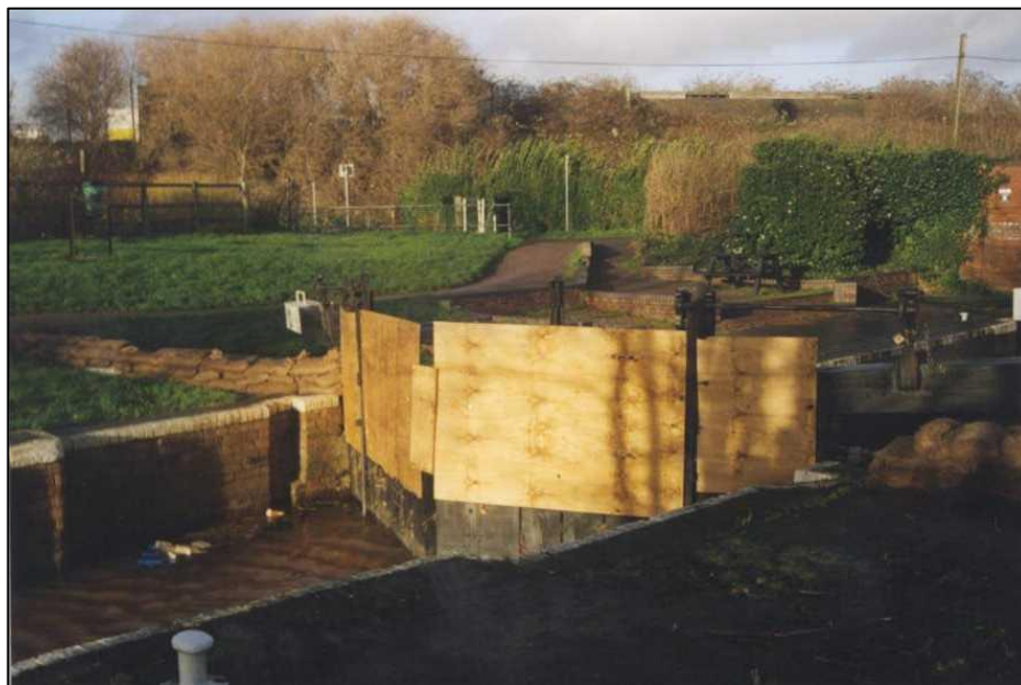
Figure 4 – Emergency works to Firepool Canal lock gates to prevent Tone water entering the canal in 2000. (Environment Agency).
